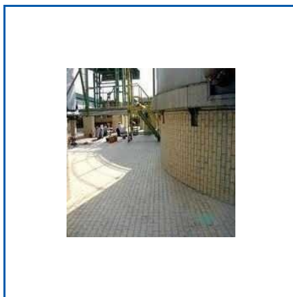
ACID PROOF BRICK LINING SERVICES
