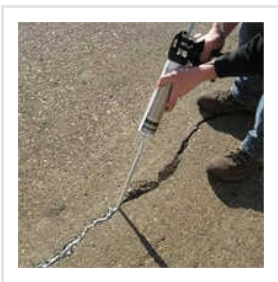
Epoxy Crack Filling Service
