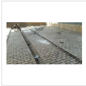
Acid Proof Tiles Lining Work
