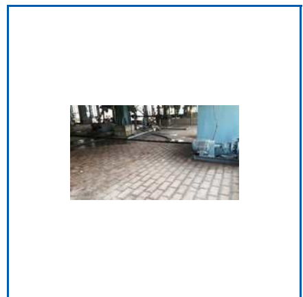
ACID PROOF TILES SILICATE INSTALLATION SERVICE
