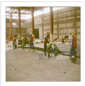
Epoxy Resin Floor Screeds
